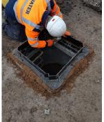
used to bed the manhole cover and frame. The surfacing was then laid to level and road was re-opened to the public.
