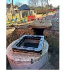
A class ii mortar was used to lay and level the TORiser units.
