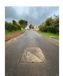
The pipe and ring were back filled to surfacing level.
